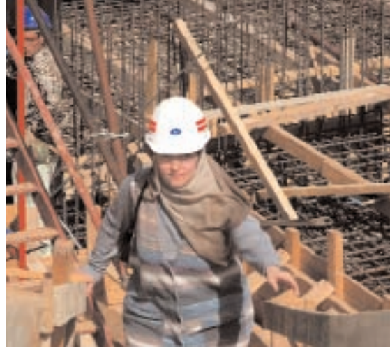
Amid the construction work on AUC's new campus project site
