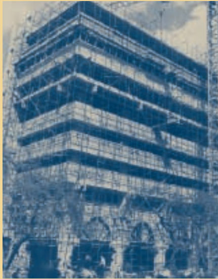
The Jameel Center in its construction phase
