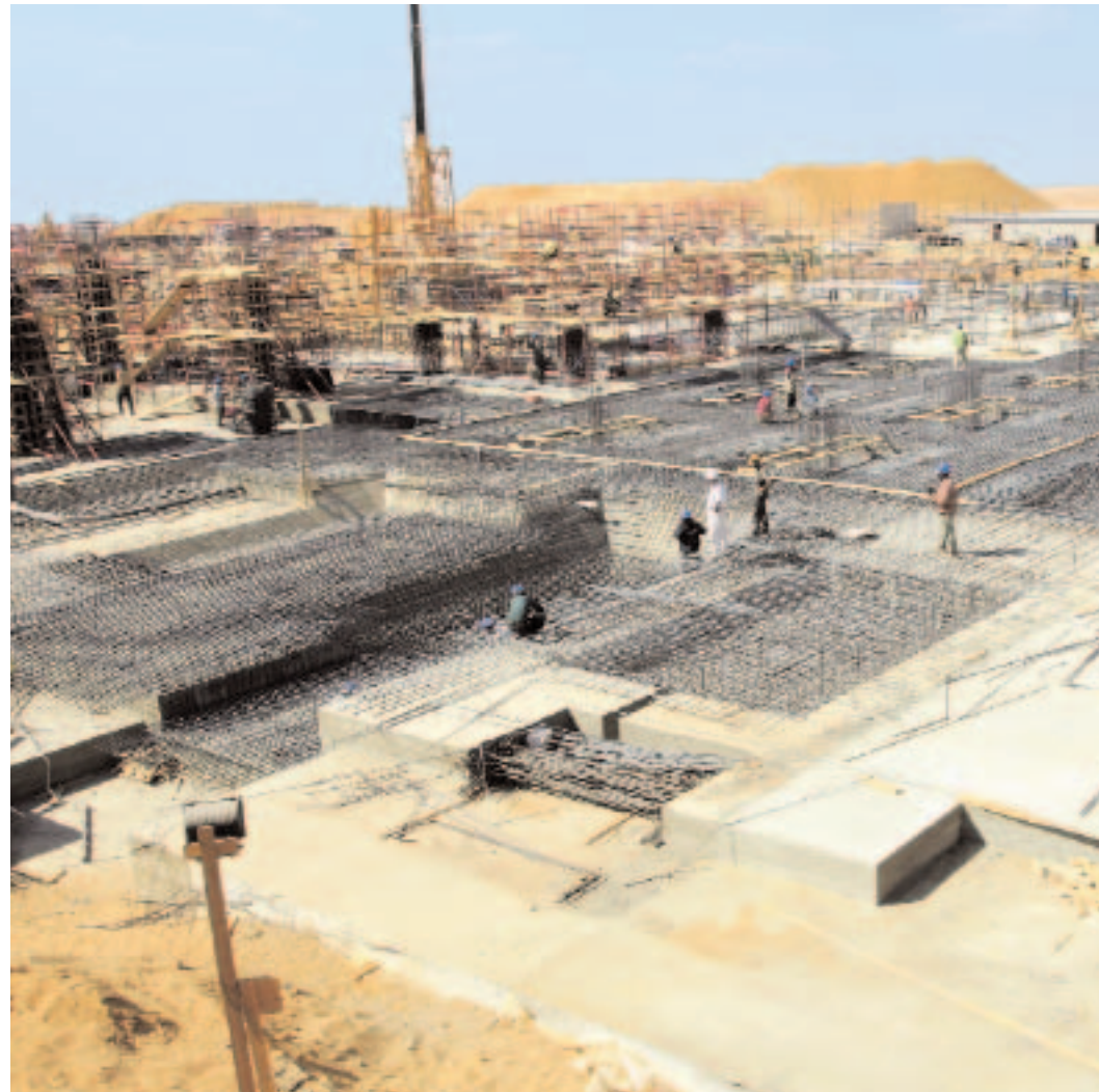
Foundation works are underway for the new AUC library
